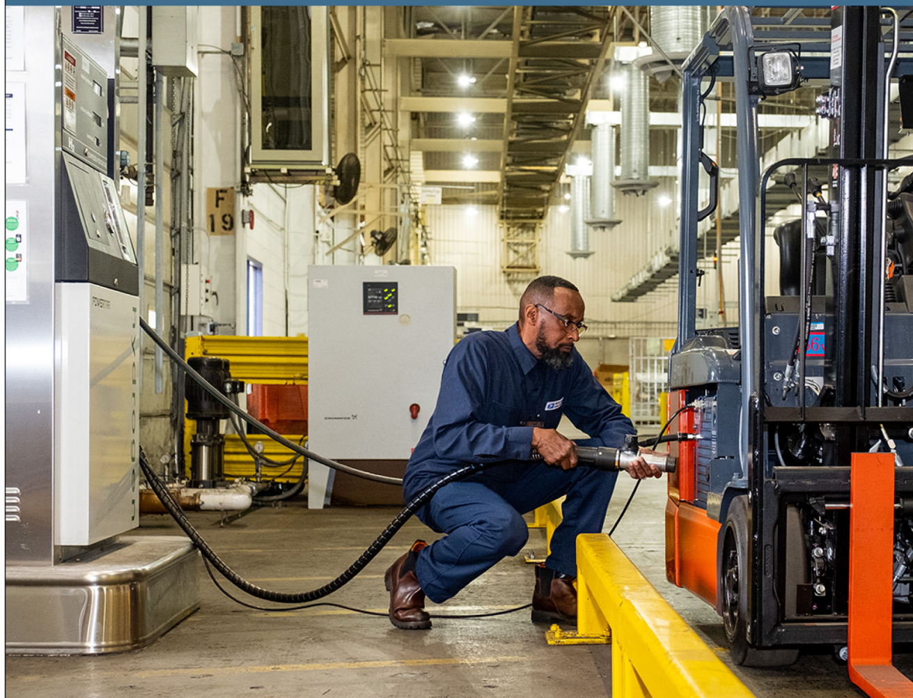
Hydrogen fuel cell powering a forklift at the USPS® Washington Network Distribution Center in Capitol Heights, MD.
